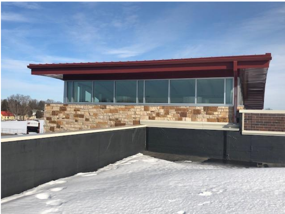
Figure 5 - Northeast Parapet Wall
