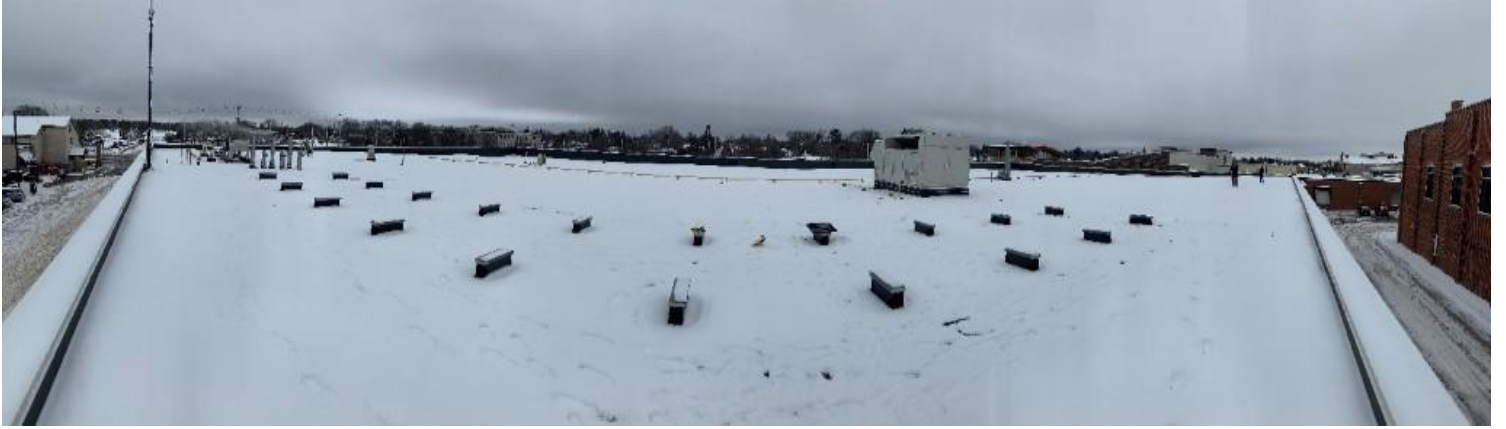
Figure 2 - Panoramic View of Roof Plane
