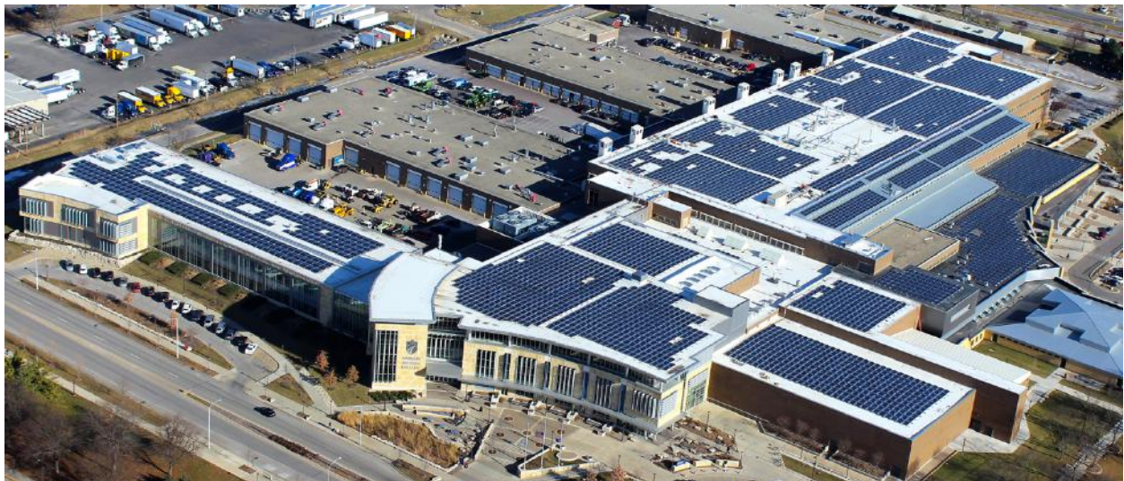
Figure 2. View of the 1.85 MW solar PV system at Madison College's Truax Campus
