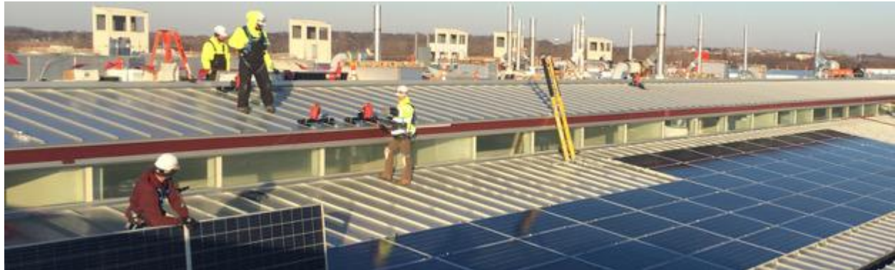
Figure 6. Photo of the Madison College solar PV system installation in progress
