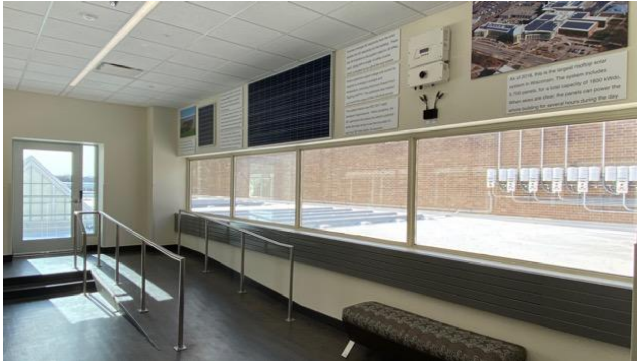
Figure 5. Observation viewing deck, roof access door, and ADA compliant ramp for the student instructional subarray for the Madison College solar PV system
