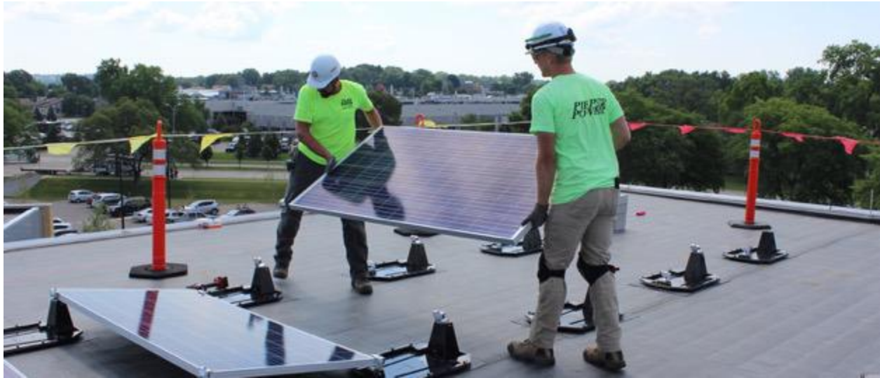
Figure 14. Madison College alumni work on the rooftop solar installation.
