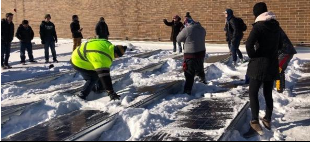
Figure 12. Students at Madison College clear snow from the instructional subarray to assess the costs and benefits of solar operations and maintenance.
