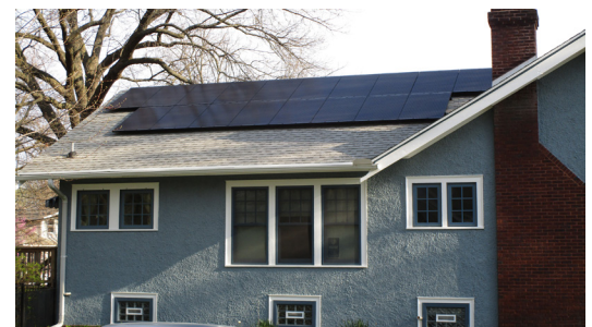
5.10kW array installed on residence as part of Solar Urbana Champaign 2.0 Group Buy.
